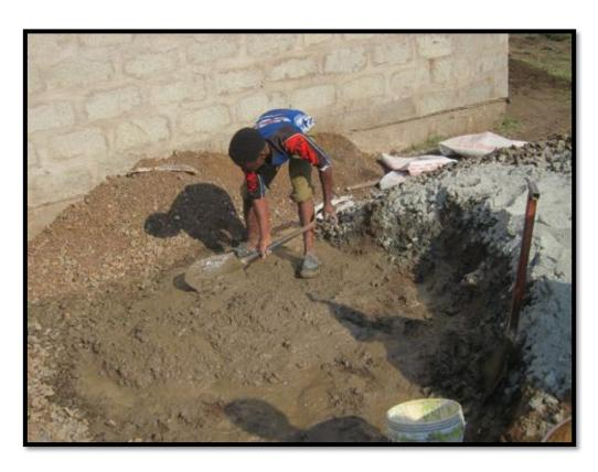
Step 4: The concrete mixture was deposited and leveled uniformly.
