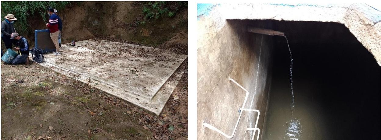
Figure : Distribution tank of 3 Parajes System.
