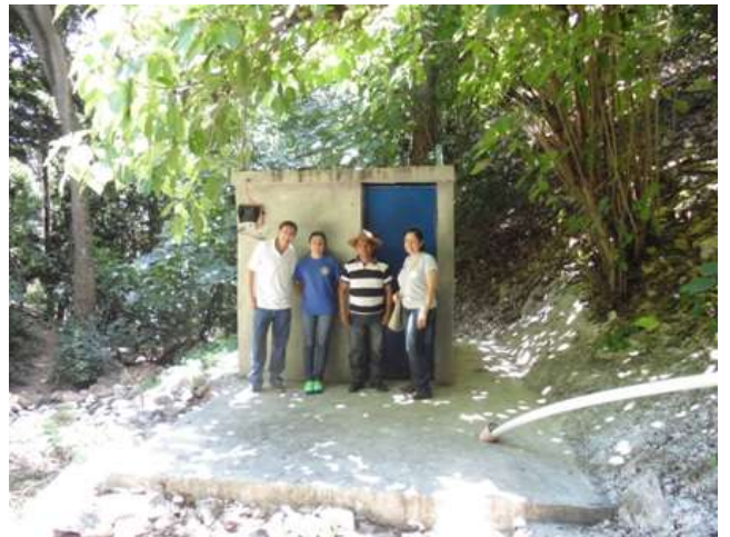
Chiquimula Rotarians Oscar, Lorena and Veronica with the head of the Los Lorenzo water board, third from left, at the completed Catchment Tank and pump house. The pump to get water from this tank to the Distribution Tank was supplied by the municipality of San Jacinto.
